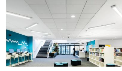
Rockfon Koral was fitted with Chicago Metallic T24 ECR grid to combat areas of high humidity. Built for challenging indoor environments, Chicago Metallic T24 ECR grid has enhanced corrosion resistance to withstand exposure to moisture vapours and temperature changes. Rockfon Koral provides 100% humidity resistance which ensures the ceiling is dimensional stability even in extremely humid conditions.
